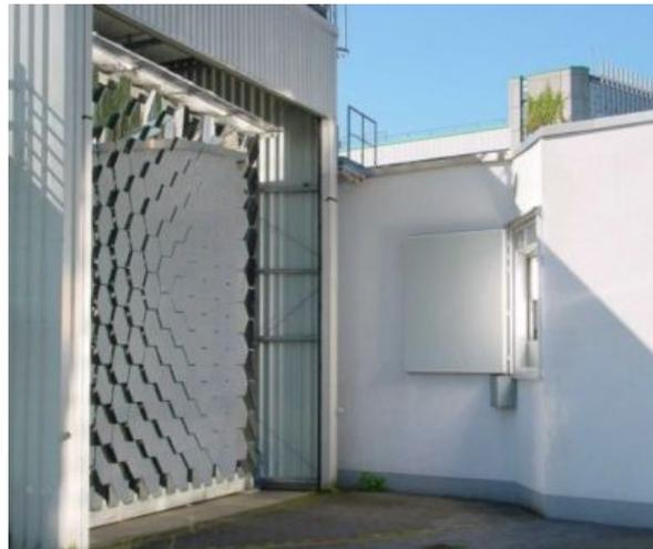
**Figure 2:** DLR solar furnace concentrator
